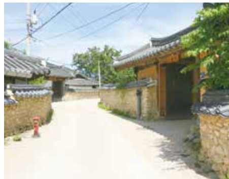
Figure 2. Layout of alleys and gates in Hwangsan Village, Geochang, Gyeong-sangnam-do province, according to the idea of chungpa .
