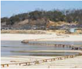
Figure 6. Single-log bridge in Museum Village.
